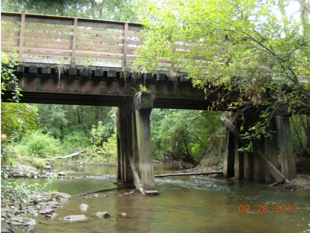
Downstream Looking West
