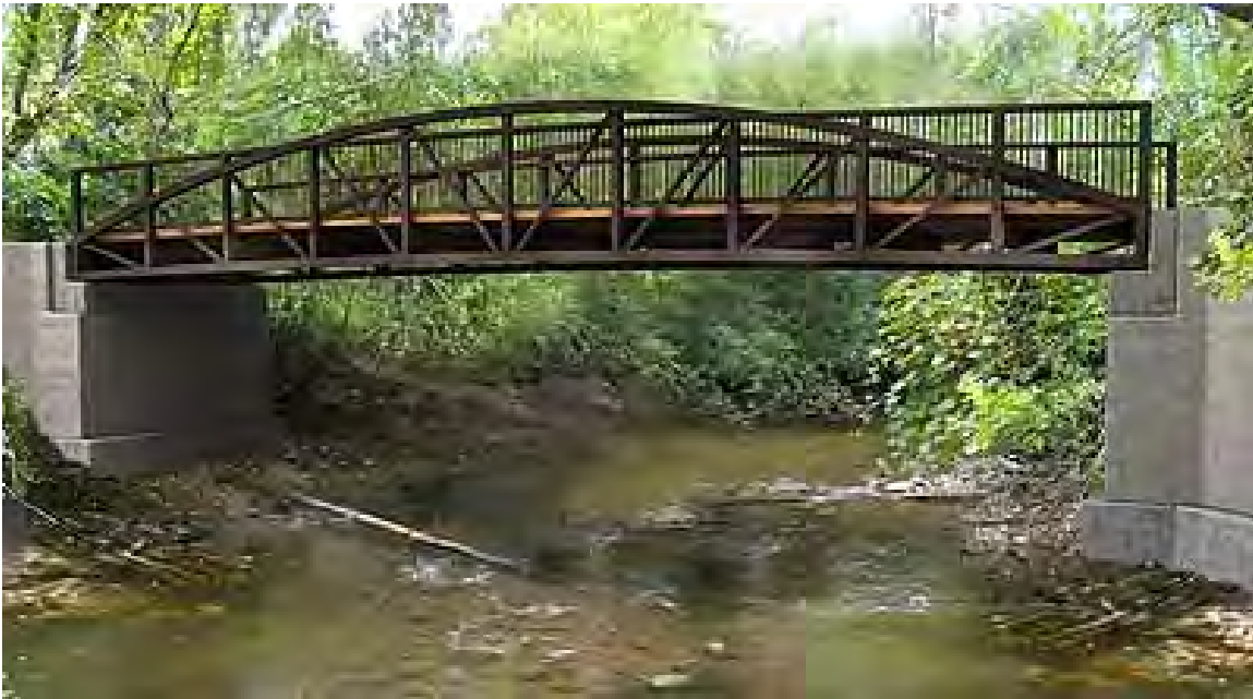
Prefabricated Steel Truss, Weathered Steel
