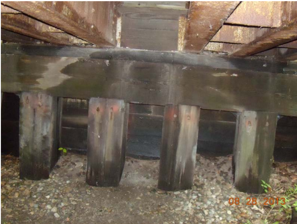
North Abutment/Retaining Wall / Pier/Bent Looking North
