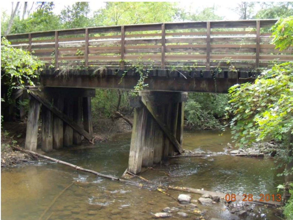
Upstream Looking East
