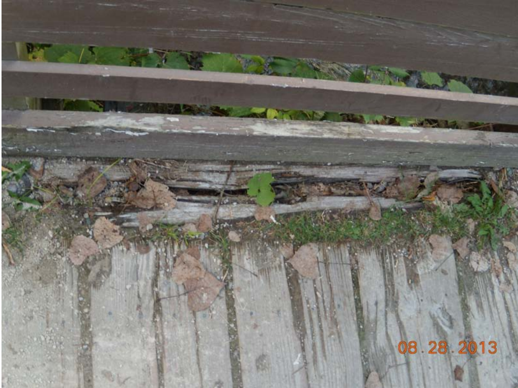
Deck Edge at Southwest Corner
