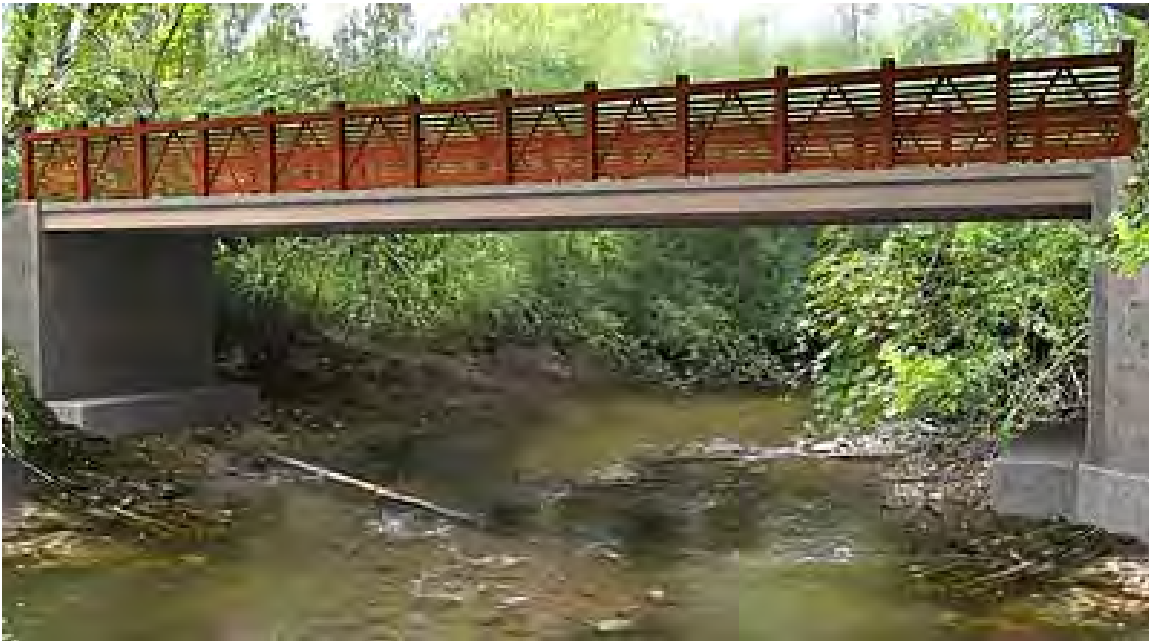
Prestressed Concrete Box Beam and Weathered Steel Railing
