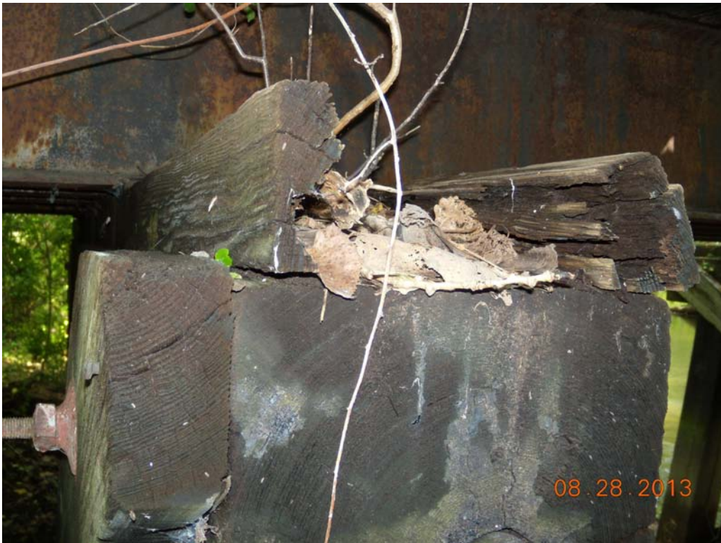
Pier/Bent Cap Second from the North, West Side
