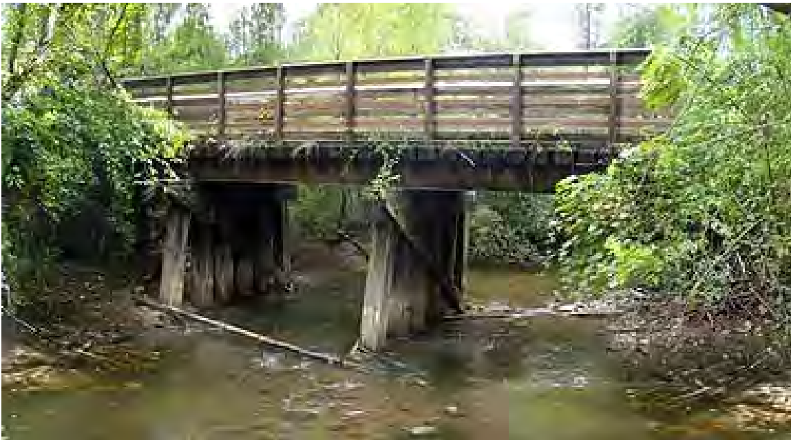
Character of Existing Bridge Relatively Unchanged with Rehabilitation
