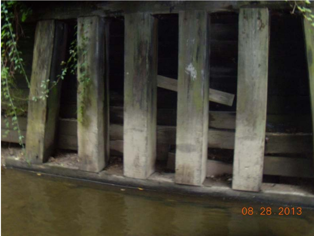
South Abutment/Retaining Wall / Pier/Bent Looking South
