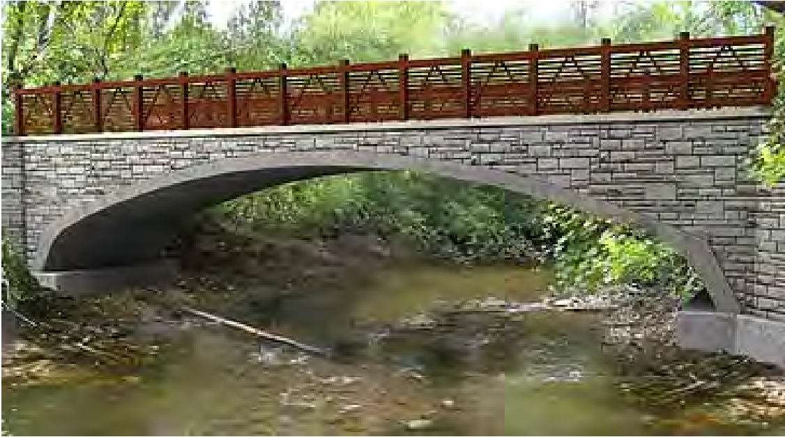
Precast Concrete Arch with Decorative Finish and Weathered Steel Railing
