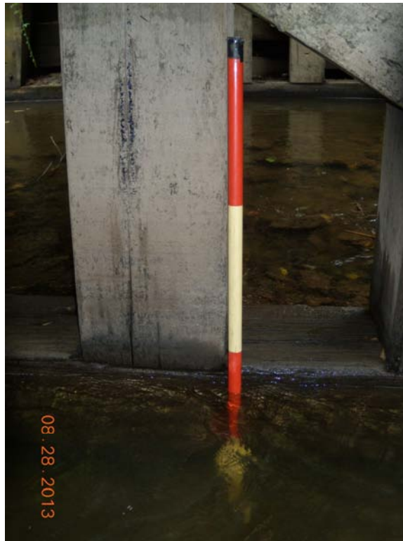
Second Pier/Bent from South Exposed Footing on North Side
